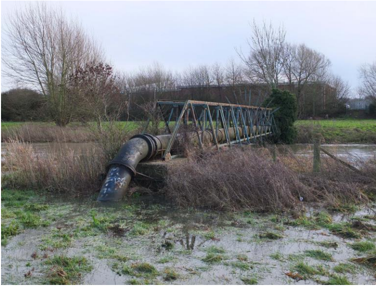
5 pipe over the Stour
